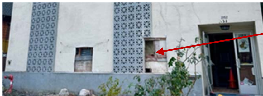
Exploratory holes made to assess the condition of the original facade.
