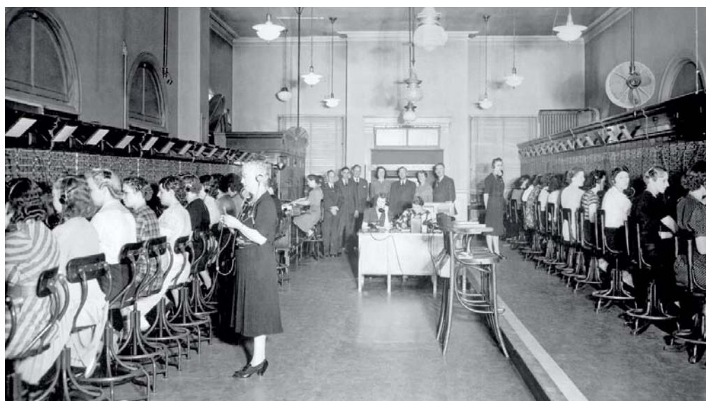
Fig. 3: Interior of the Sunset Telephone Exchange, sometime in the 1930s.
