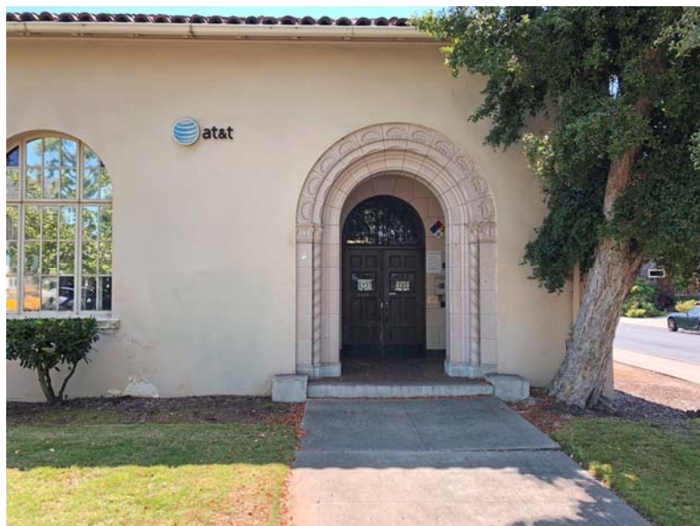
Fig. 6: Part of the building down the street at 2100 Central Avenue, which replaced the switchboard in the old building around 1940. It remains an AT&T facility today.
