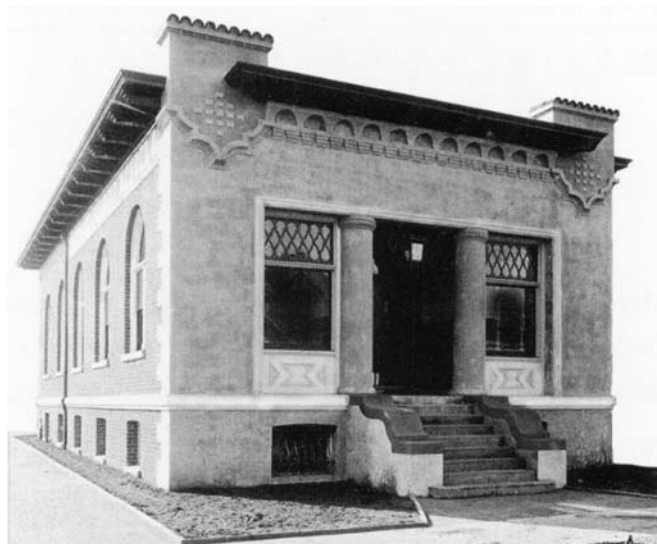
Fig. 2: The Sunset Telephone Exchange at 2152 Central Avenue in Alameda, showing original facade. A project is underway to restore facade to its original ornate appearance.
