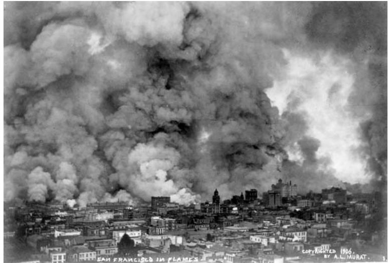
Fig. 5: Fires following the 1906 San Francisco earthquake. Library of Congress photo.
