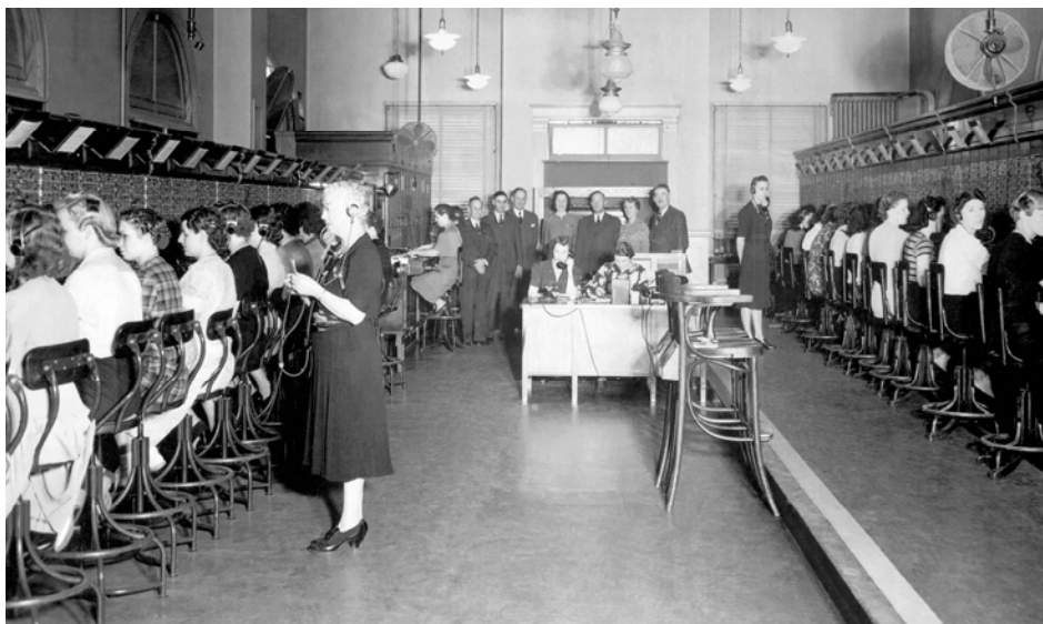
Telephone switchboards were the original use for the CHRS RC building in Alameda.
