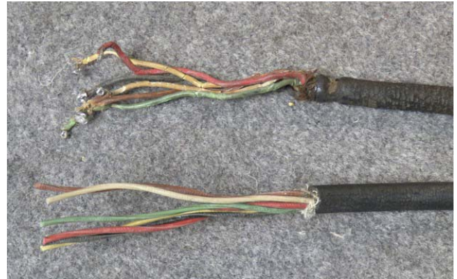
Cable ends trimmed and repaired.
