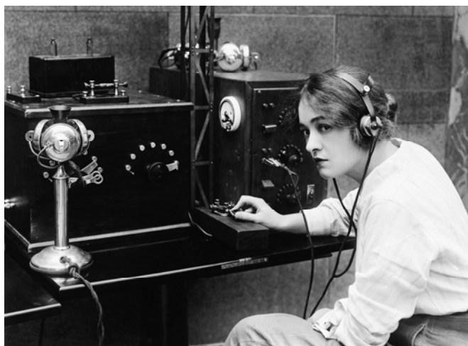
The props include on the left an induction coil and in front of it a spark gap and to the left of that, a condenser for headphones. The large box may be meant to be a switched capacitor for a transmitter. The microphone or telephone is of an odd configuration. The lady works a key. Her headphones connect to a receiver with a rheostat (for filament voltage control) at its side. More headphones sit atop the receiver. A central tower guides the antenna lead.
