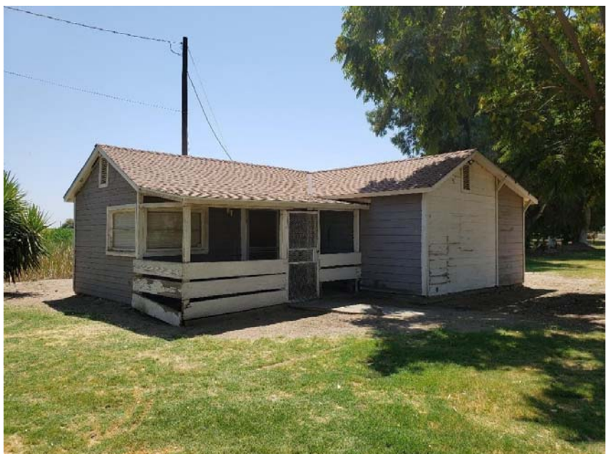
The Central Valley Chapter clubhouse with a new roof.
