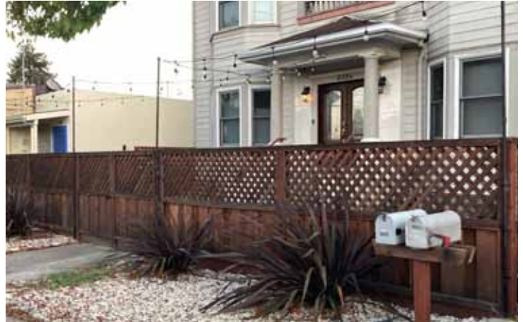
5' tall fence that does not meet the City's current transparency requirements and obstructs the front of the house.
