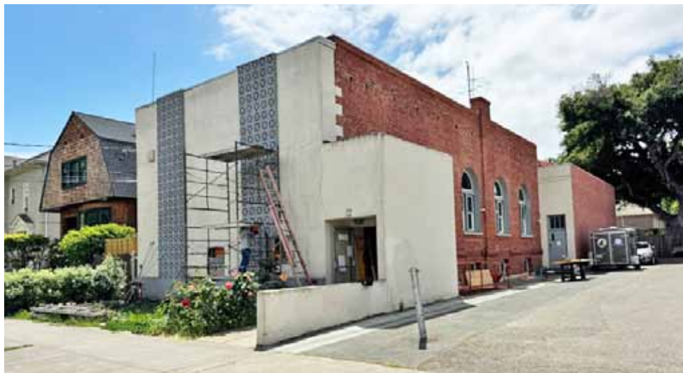
2152 Central Avenue with the false front in April 2024.
