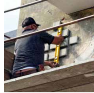
Raised ornaments are carefully measured and attached.
