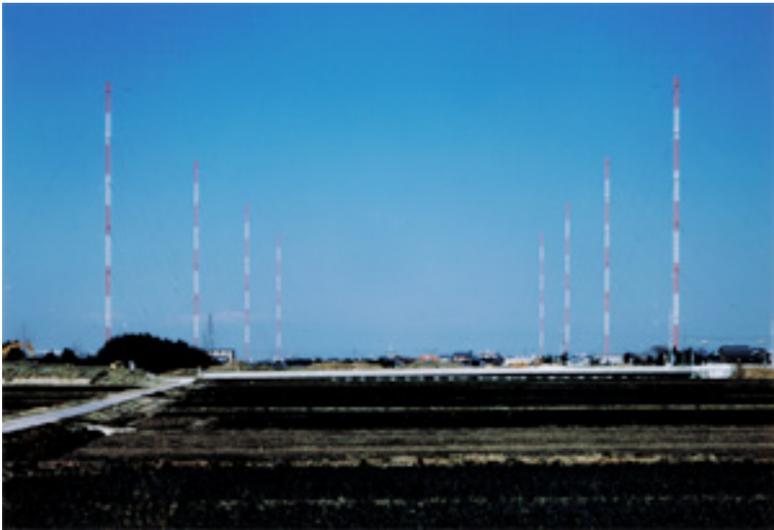
The VLF Towers
