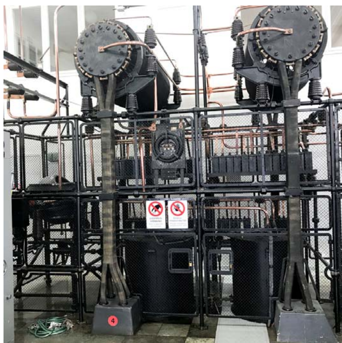
Fig. 7: Output circuits to the antenna.
