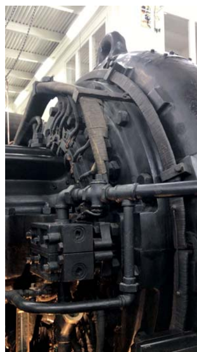
Fig. 8: Thick cables connect the alternator to the tuner.
