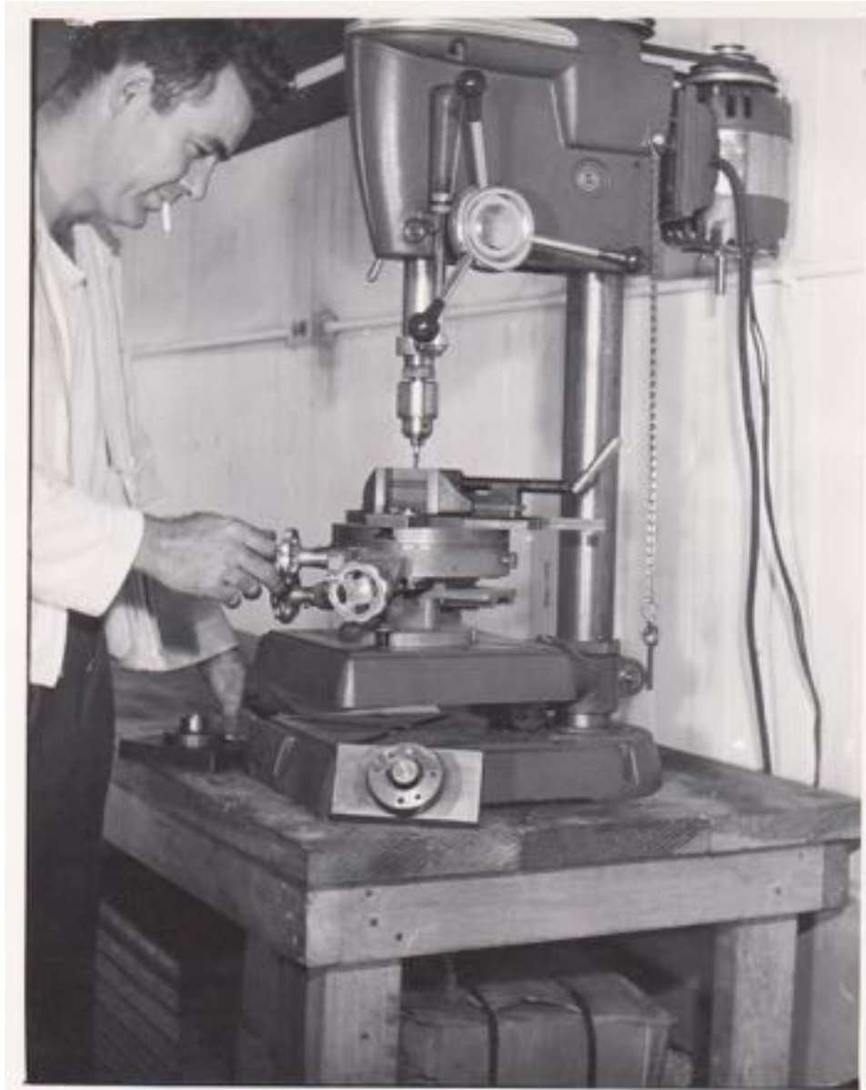
A Drill-Press Adapted as a Vertical Mil
