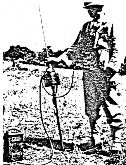
SCR-511, designed for cavalry in 1940, was the only light Walkie-Talkie when WW II broke out, and saw wide use by infantry.
