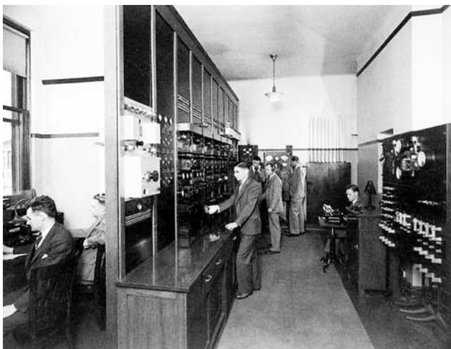
Left: Master Control at NBC in San Francisco, used from 1927 to 1942 with studio amplifiers, bridging equipment, power and testing equipment.
