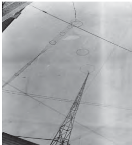
Figure 8. Bart Molinari's 6AWT cage antennas; photo from C. West 5CN album (author's collection).
