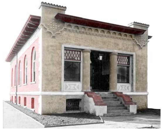
Original circa 1900 exterior front elevation of 2152 Central Ave.
