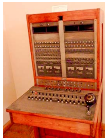
Fig. 6: A later switchboard.
