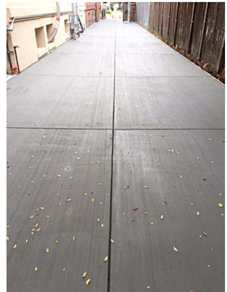
Newly poured driveway.
