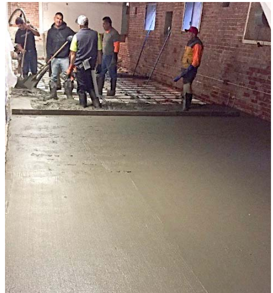
Pouring the downstairs floor.
