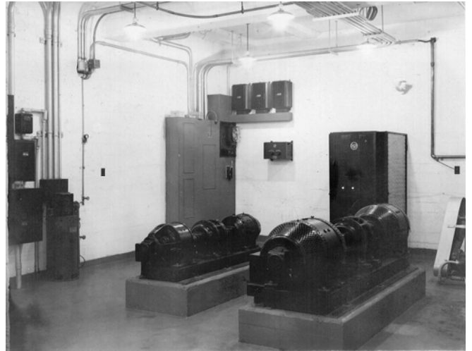
KYA generator in the basement, 1937.
