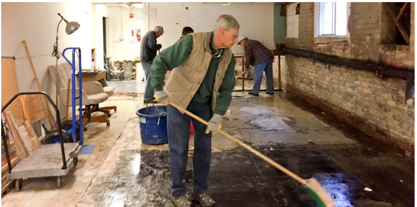
Denny, Hill, Dave, and John removing water from the flooded basement. An ongoing job as the water repeatedly flowed in when it rained — which, last winter, was often.
