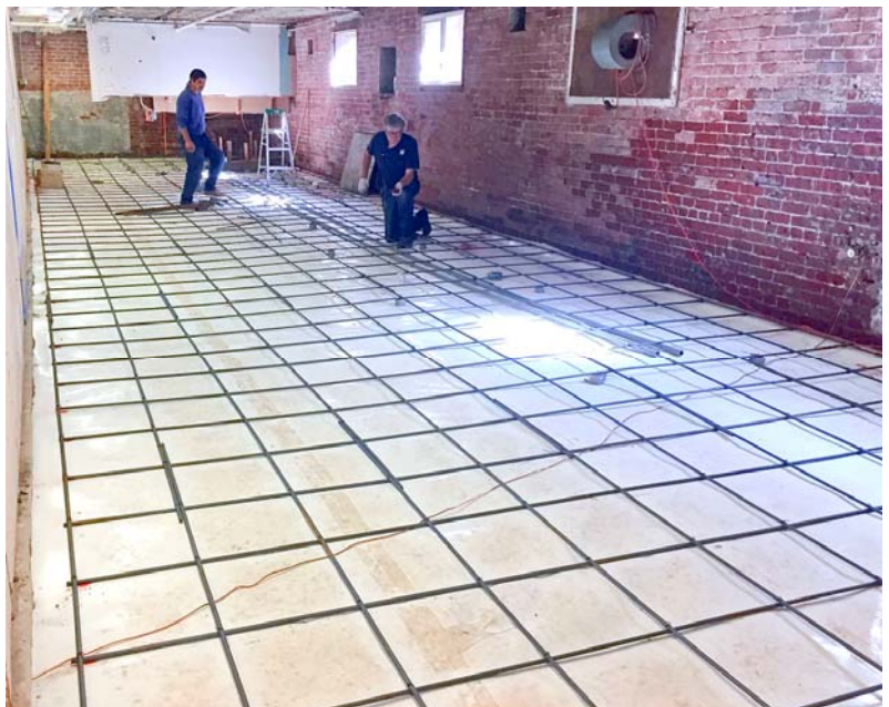
The downstairs floor progress at the time of this journal printing. The old floor was removed, drain trenches were dug, and the area covered by a thick layer of gravel. Then the thick white Preprufe covering forms a waterproof barrier. Next the rebar grid will be raised on dobies, and then the pour of the 6" thick concrete floor. The brick walls were sandblasted.
