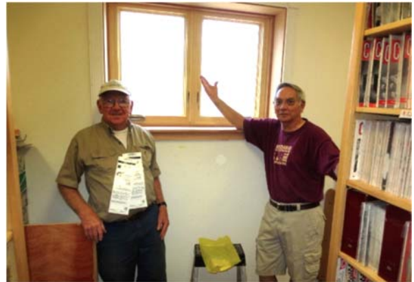
Larry Drees and Robert Swart finish installing a new window.
