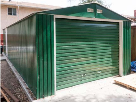
Newly constructed Wood and Crafts Shop.
