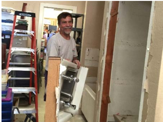
Keith Scott removes an old sink.
