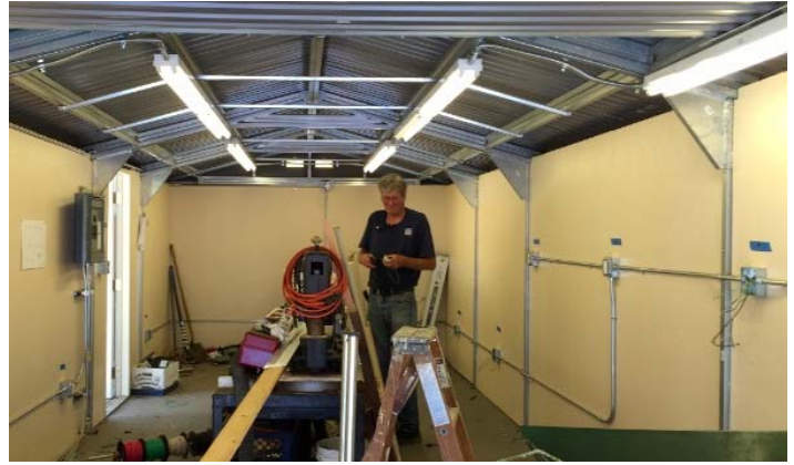
Kevin Payne installing electrical in the wood and crafts shop.
