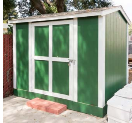
Refurbished garden shed.
