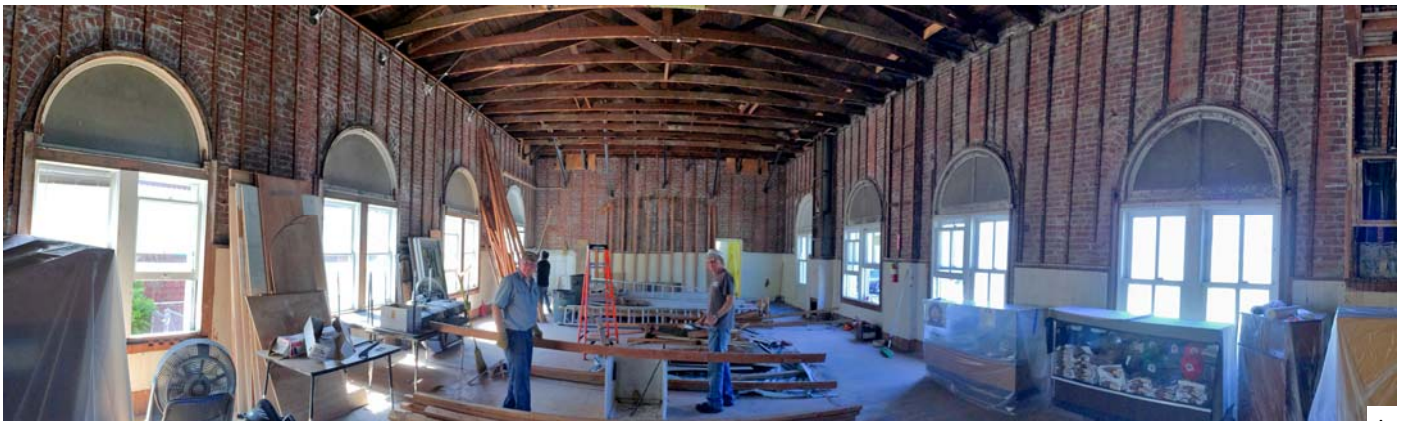
Main room after plaster and church sanctuary walls at far end were removed. Photo by John Stuart.
