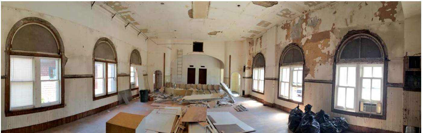
Main room after T-bar suspended ceiling, soffits, and asbestos popcorn wall and ceiling insulation were removed. Photo by John Stuart.
