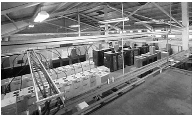
Transmitter gallery in Building 2a. Vintage 1950s vintage RCA plus 1990 vintage Henry transmitters. Source MRHS Point Reyes
