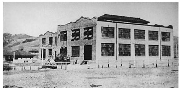
Marconi transmitter building (Building 1) and cottage 1 (circa 1920). Source MRHS.
