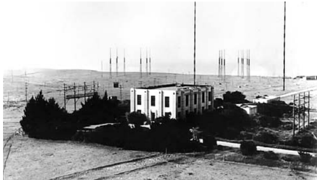
RCA transmitting building (Building 2) constructed in 1931. The two 300-foot antennas visible behind (1940s). Source MRHS.
