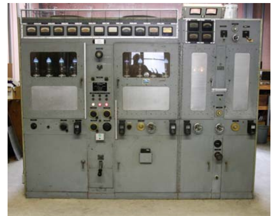
The Press Wireless PW15 transmitter in operation in Bolinas Building 2A.
