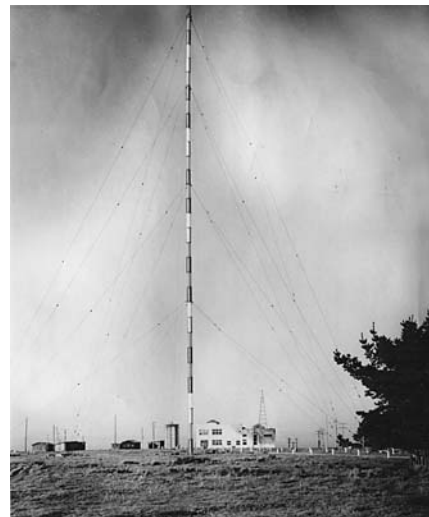
Marconi transmitter building and one of the 300' Marconi towers. By the 1940s the towers were painted alternating colors for visibility (1951). Source MRHS.
