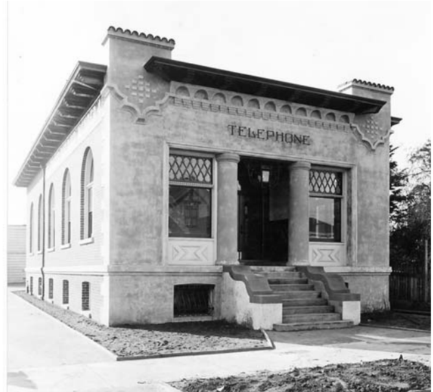
Original exterior front elevation of 2152 Central Ave.
