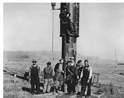
Riggers working one of the 300' Marconi towers (1930s). Source MRHS.
