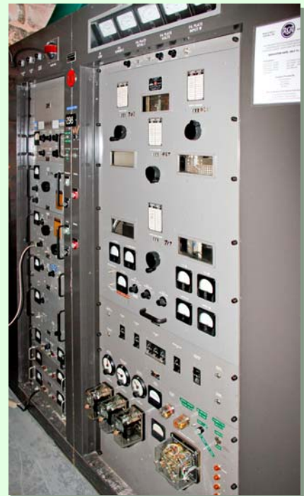
Front view of the restored RCA transmitter. ◇
