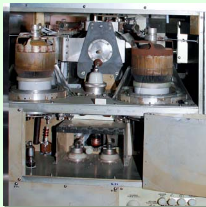
'After' condition: Restored interior of the RCA transmitter.
