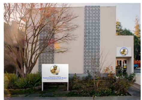
2152 Central Avenue in Alameda, CA.
