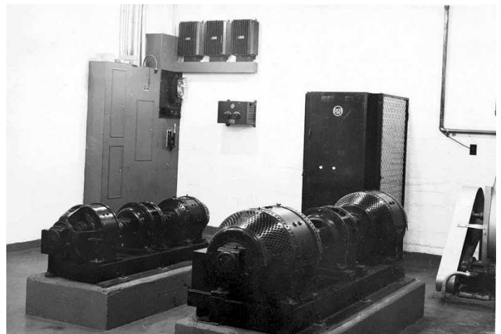
Fig. 22: Generators in basement of new transmitter building.
