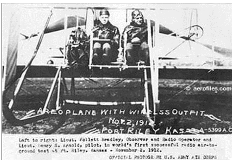
Fig 3: Airplane with wireless outfit 1912 (Left) Observer and radio operator, (Right) pilot. Source: Aviation time line chronology—Aerofiles.com
