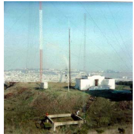
Fig. 40: Replacement antenna tower (1987).
