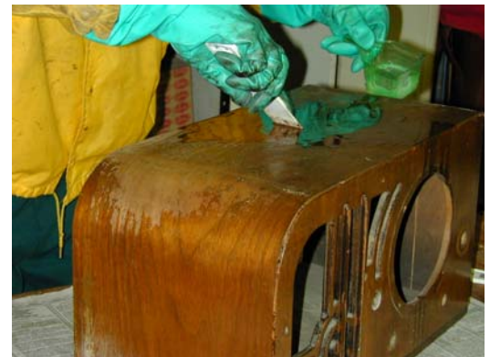
Figure 8: Stripping the softened old finish with scraper and lacquer thinner.
