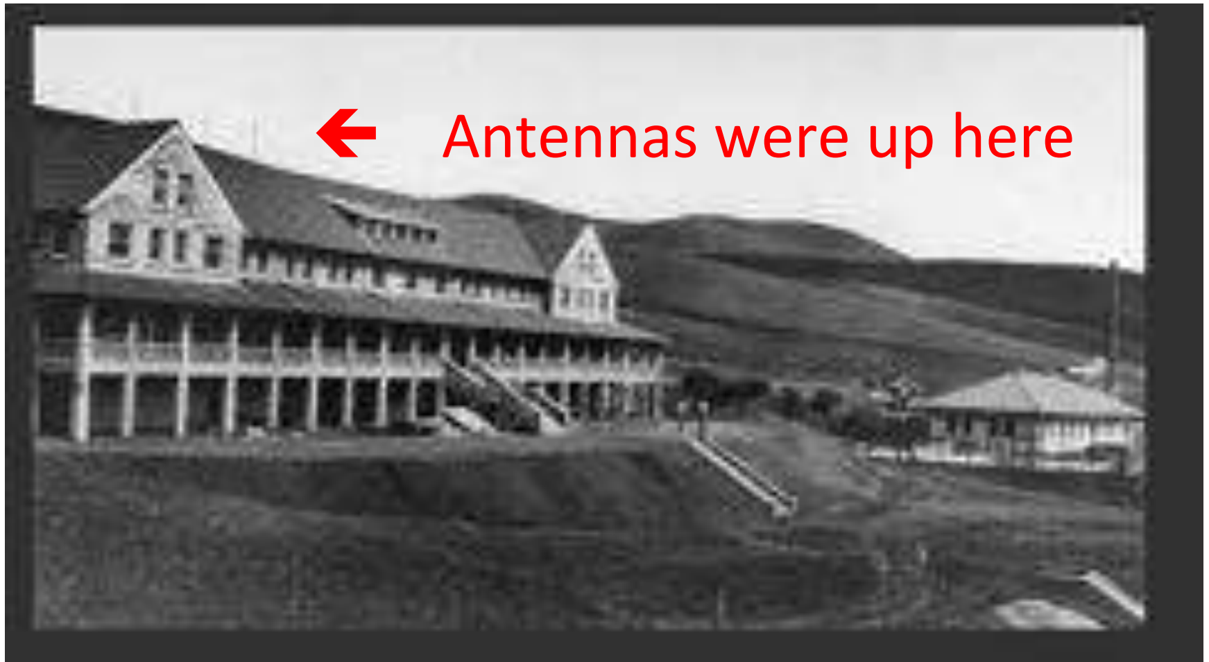
Antennas were on the Hills; 1914 Marconi Operators Hotel (“de Gink”)
