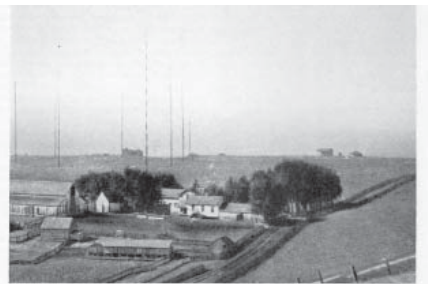
Fig. 35. The Bolinas, California American Marconi station low frequency antennas in 1917. The 1920-21 KEI alternators used a different antenna system of a line of radiating vertical towers with long lines of wire between them acting as a high capacity “hat” to permit very low frequency operation in the range or 15 KHz.
