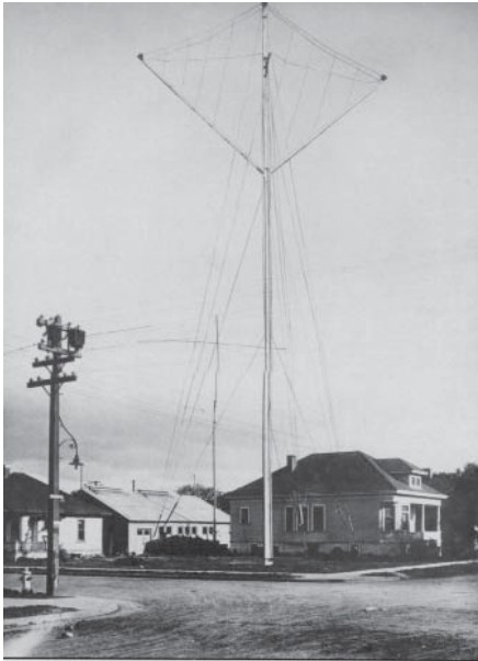
Fig. 27. The genesis of the Cyril Elwell and Lon Fuller’s world-wide Federal arc enterprise: Amateur wireless operator Douglas Perham’s garage next to his Palo Alto, California house (the first “Silicon Valley Garage”). Later the company used all of this property. Lee de Forest did his 1911-13 Audion development work here. Perham worked for Federal and later established the Perham Collections of early wireless and radio artifacts, maintained with the support of David Packard and other industry leaders, now part of History San Jose. (Photo in Perham Collections, History San Jose)
