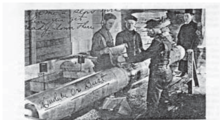
Fig. 11. A.J. Krenke and the Pacific Wireless crew constructing transmitter equipment (a large helix) about 1906 for the projected Hawaii circuit (SWP).
