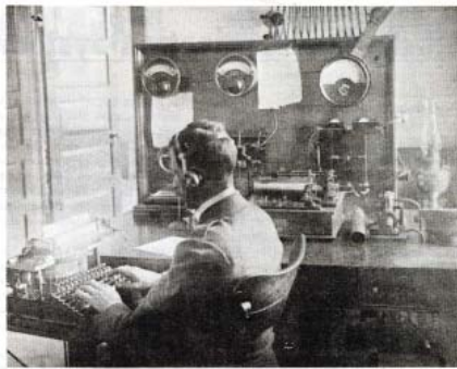
Fig. 8. Alaska Station FK about 1905 (SWP).
