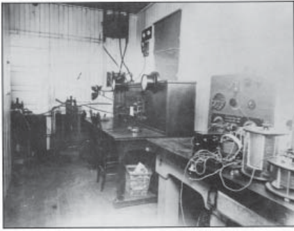
Fig. 17. The Federal Beach Station, interior, 1910; the first big arc in service (12 KW). (Mayes).
